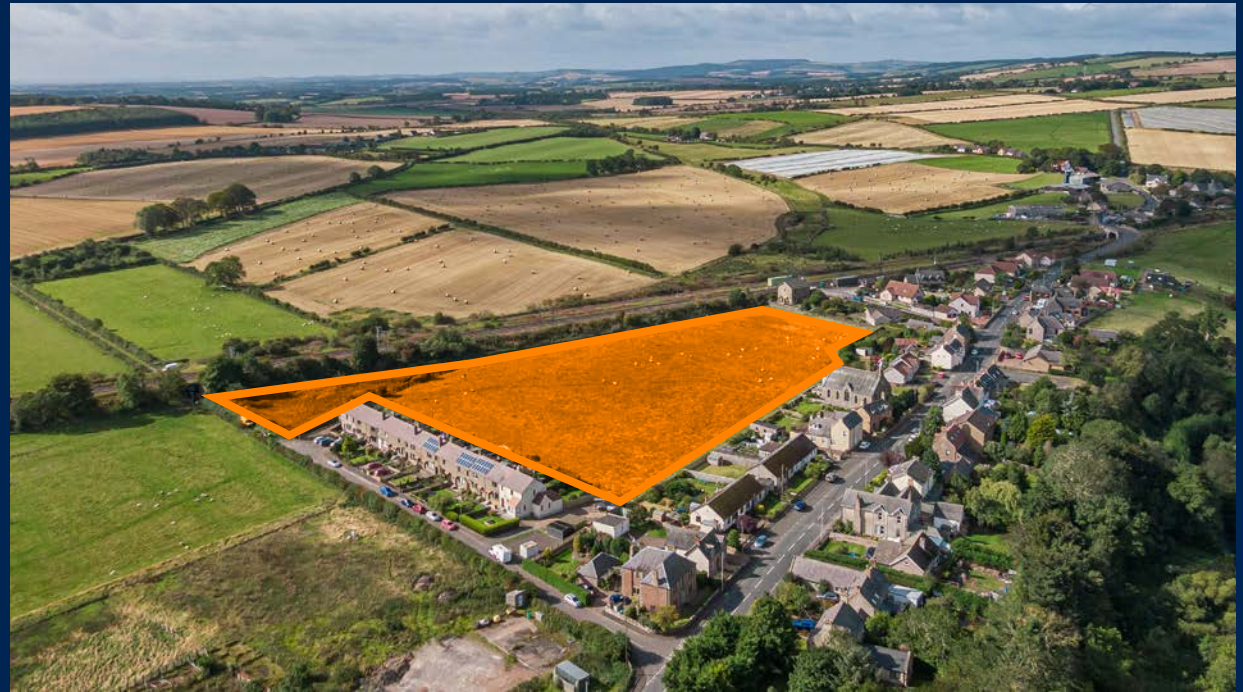
Note: Photographs taken August 2020
